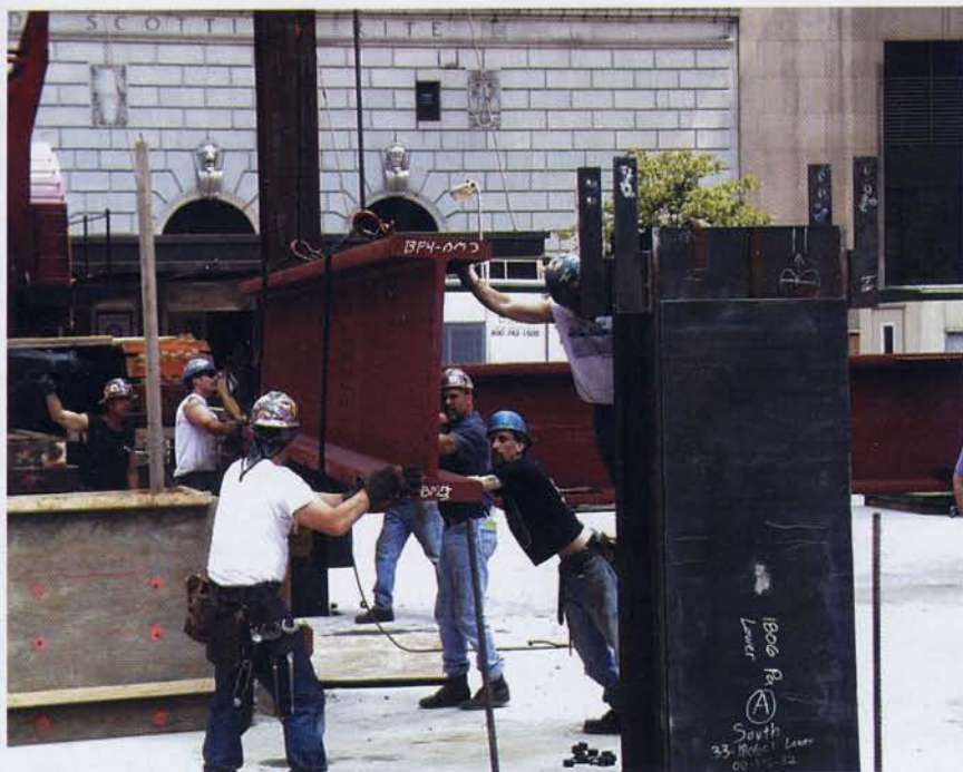
TOP: An aerial view from 34th Street. LEFT: Workers maneuver megacolumns and steel beams to construct support for a crane.
