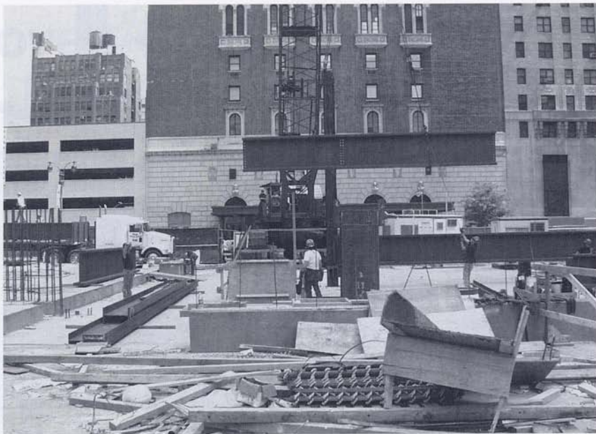
Steel beams being installed to support a crane.
