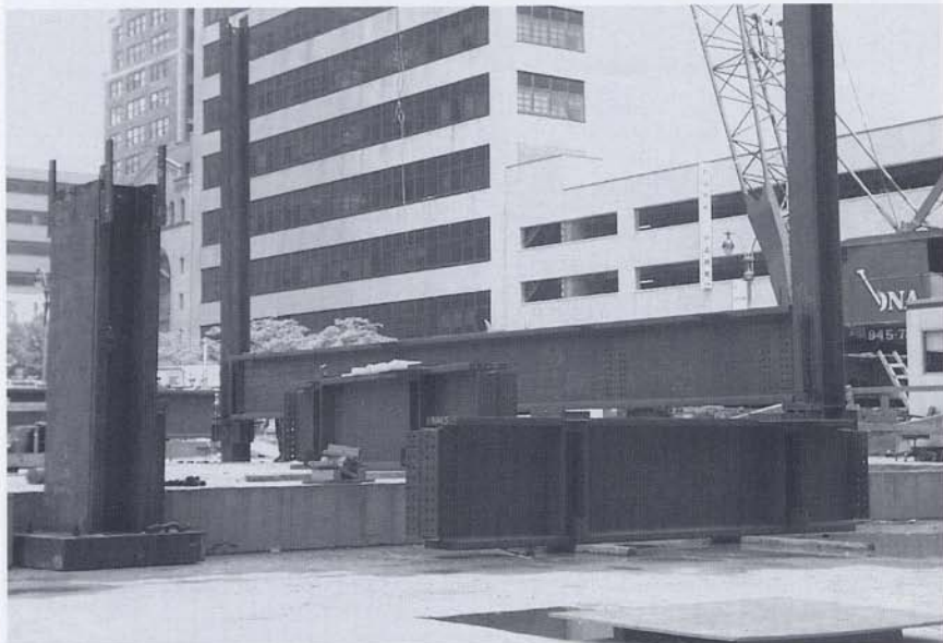
Steel megacolumns used in this project.
