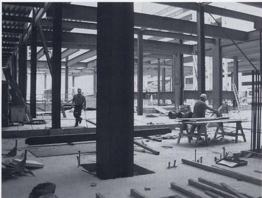
The steel structure installed above the concrete structure.
