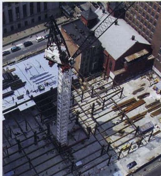
TOP: An aerial view from 34th Street. LEFT: Workers maneuver megacolumns and steel beams to construct support for a crane.
