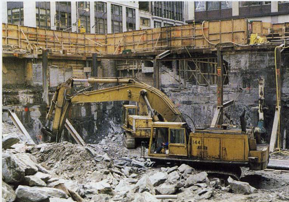
Foundation excavation looking at southeast corner of site.
