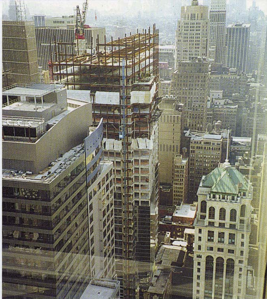
View of the north side elevation looking south.
