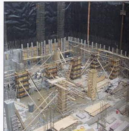
Photo: Courtesy of DeSimone Consulting Engineers
