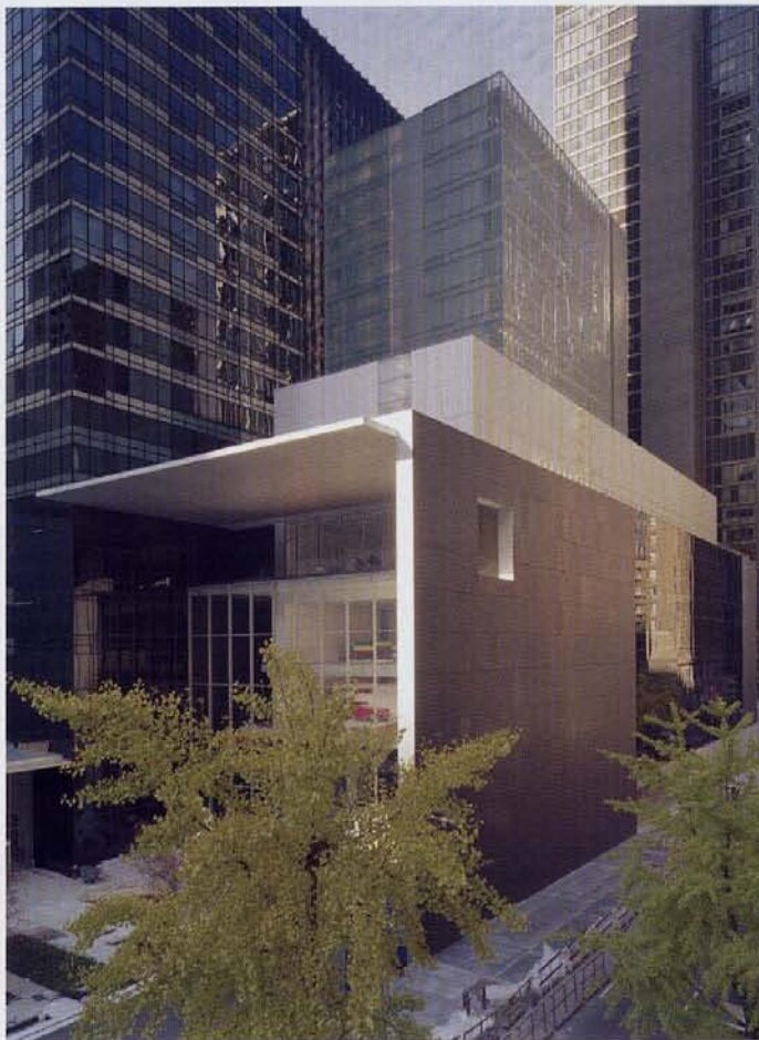
OPPOSITE The minimal stick work of the lobby curtain wall is painted structural steel.
