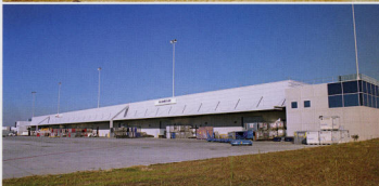
The two buildings used a total of 2,400 tons of A-572 Grade 50 steel.
