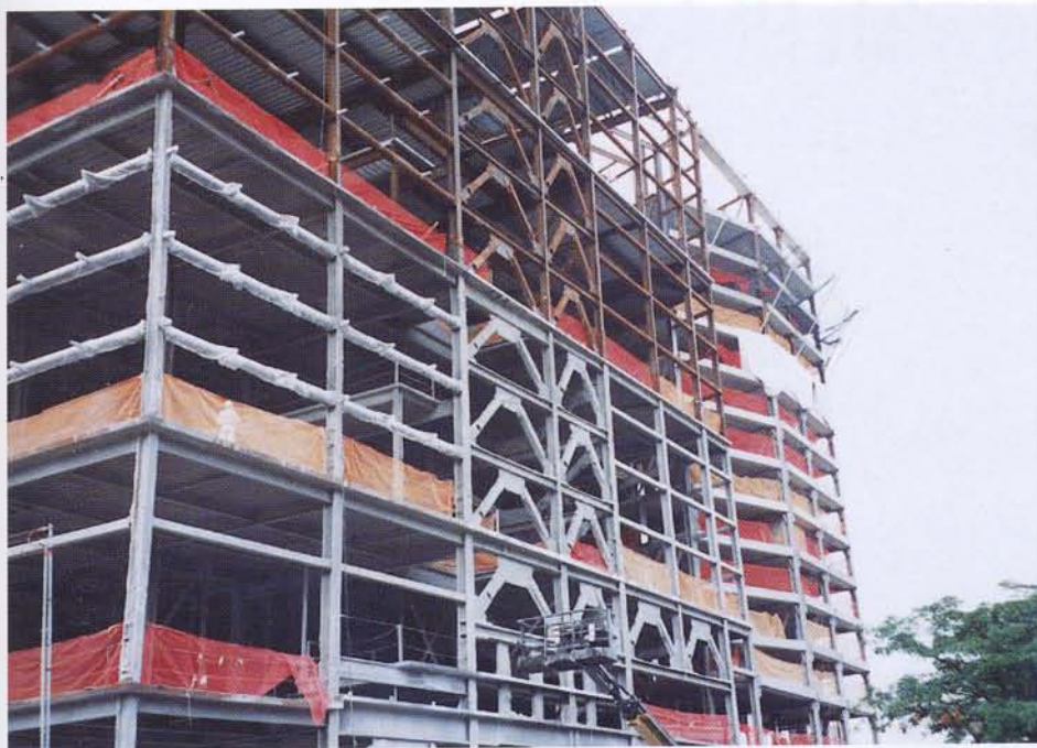
Spandrel moment frame Photos: Courtesy of Thornton Tomasetti Engineers
