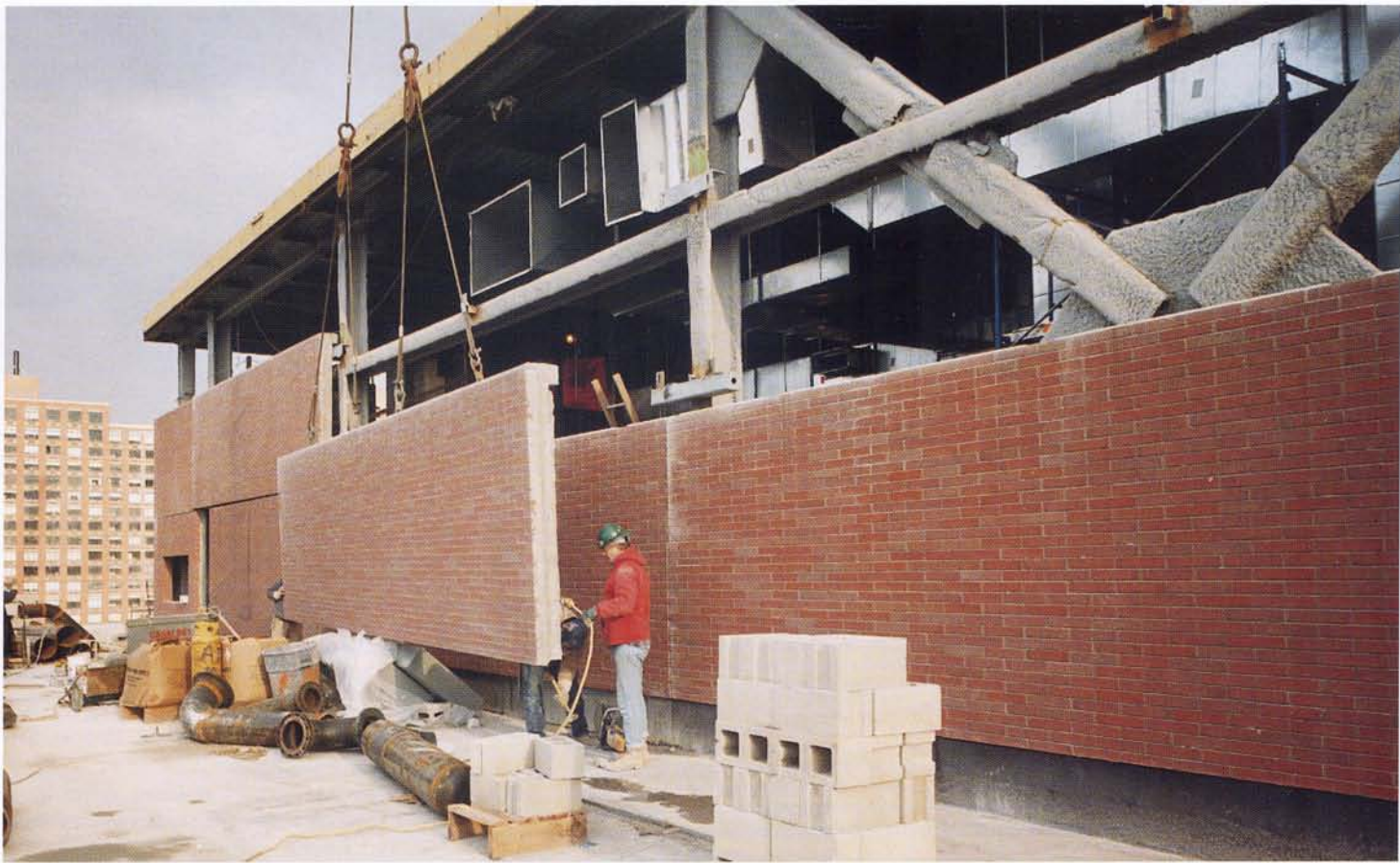
Erecting brick panels
