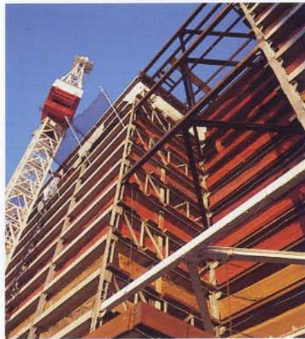
Staggered trusses Photo: Fran Soloman
